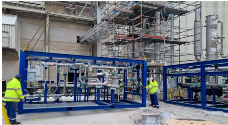
The Company’s modular membrane-based carbon capture technology enabled the plant to be prefabricated offsite and transported to Höver for final assembly. The process modules were fabricated and assembled by Blackrow Engineering in the UK and will be integrated with other equipment manufactured in the UK, Germany, Netherlands, Belgium and Italy. Blackrow’s site team are assisting Cool Planet with the assembly of the plant.
