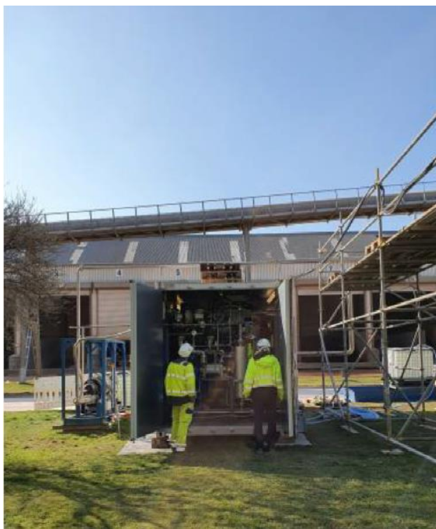
CO 2 separation plant in the Höver cement works - based on an innovative membrane technology
