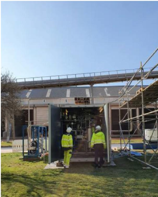
*CO<sub>2</sub> separation plant in the Höver cement works - based on an innovative membrane technology*
